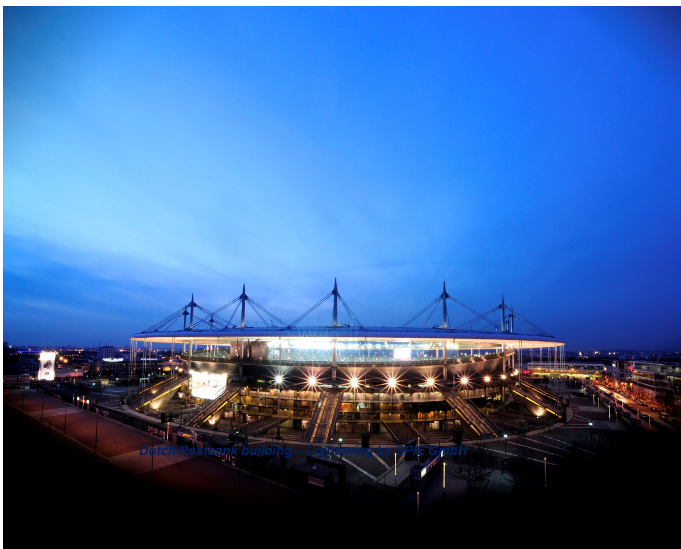
Network infrastructure in the Stade de France – Paris Saint Denis stadium - Smart City project
