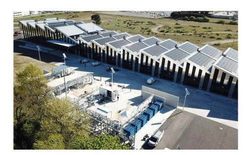
Operating autonomously thanks to a remote control system, this center is designed to reproduce real-life fuel cell operating conditions. It enables fuel cells to be tested to guarantee their robustness, quality, safety and performance before delivery to customers. This international training center is already welcoming its first potential clients.
