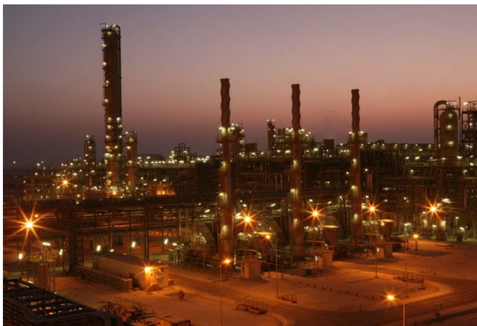
Ras Laffan Olefin Cracker Copyright: RLOC
