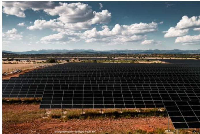
Valdecaballeros (11.4 MWp in Spain)
