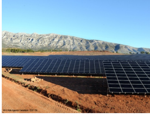
Puylobier (6.5 MWp in France)
