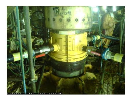
**Legend:** 25 April 2012 - A diverting sleeve has been installed on the G4 well. Known as a "diverter", this specially manufactured piece of equipment connects to the wellhead and diverts the flow of leaking gas, via four flexible hoses, away from the wellhead and the platform. This key piece of equipment improves the safety of the well intervention operation by avoiding the possibility of gas accumulating in the work area around the G4 wellhead and the platform.
