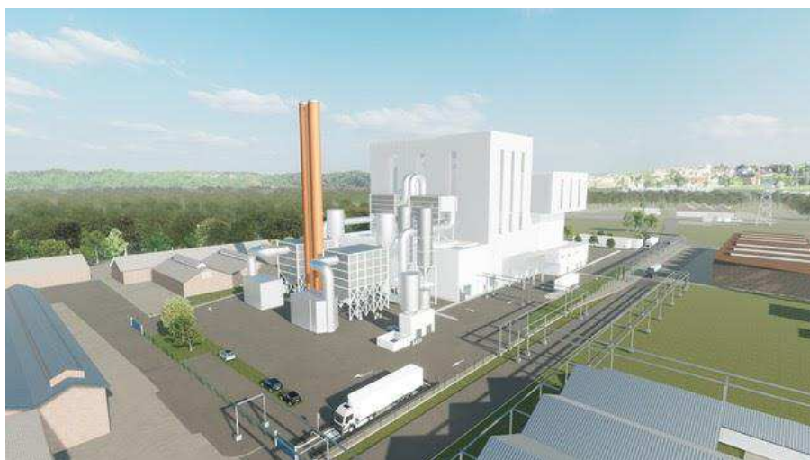
Aerial view of Solvay's plant in Dombasle-sur-Meurthe
