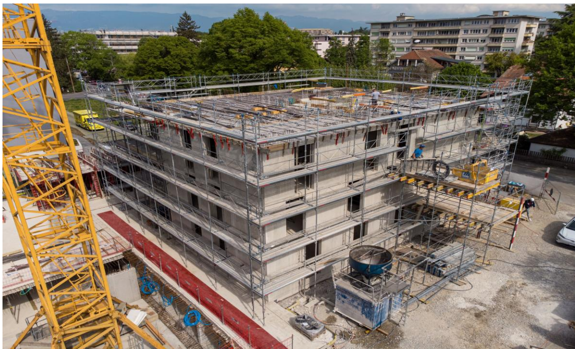
Rambosson building site of 18 flats in Geneva (Switzerland)
