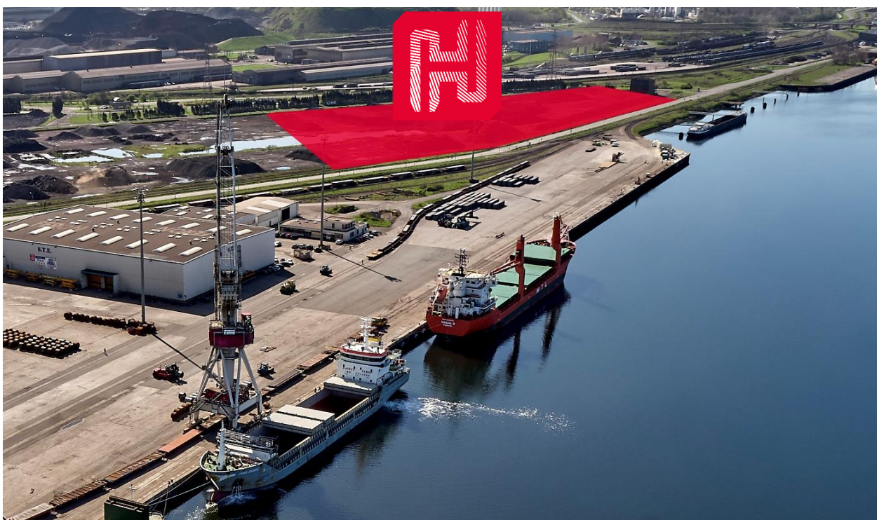
The land where the third production site (H3) will be built in the port of Dunkirk Photo credit: Dunkerque-Port
