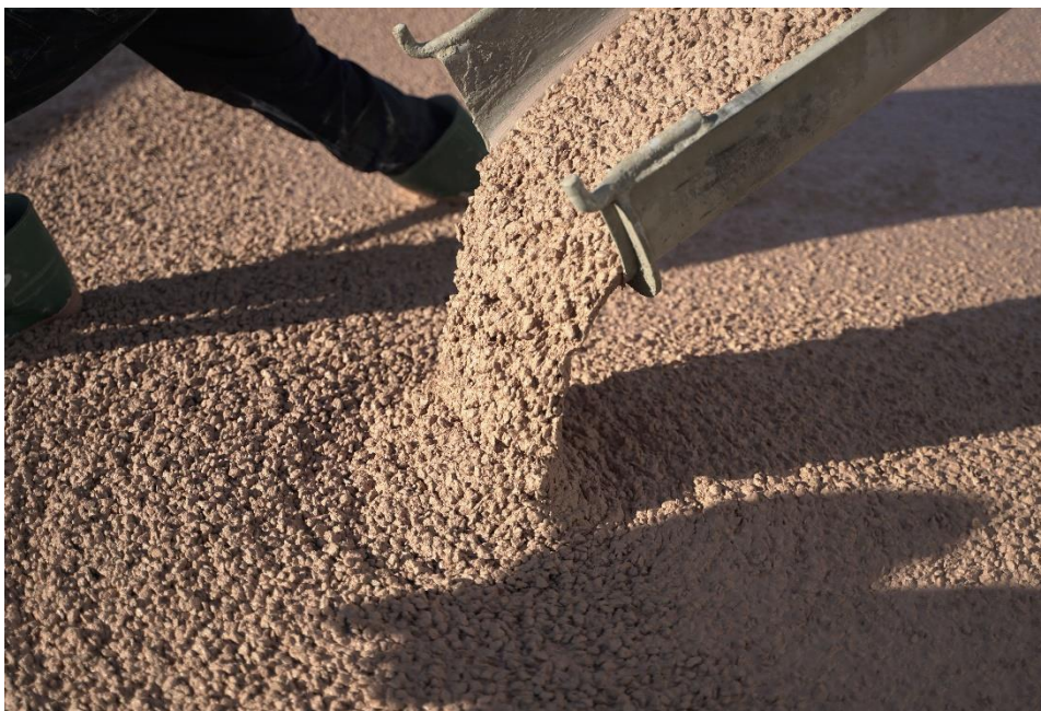
Pouring a slab of H-EVA clinker free and low carbon concrete
