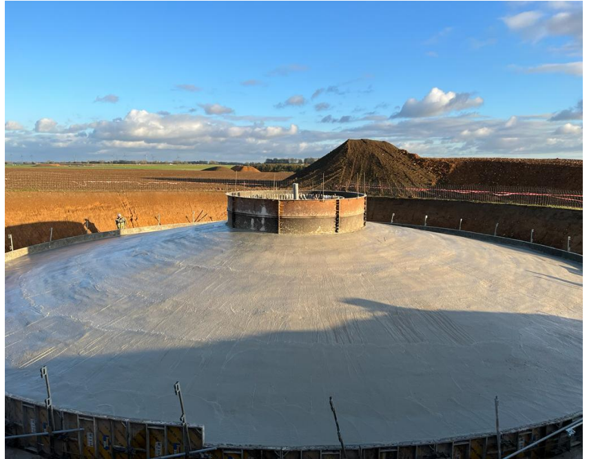
Wind turbine foundations made by Fondéole Group
