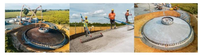
On the site of the Plaine des Moulins wind farm in Jazeneuil (Vienne), the VALOREM Group wanted Hoffmann Green and its partners to achieve a world first: the pouring of a wind turbine foundation using 630 m3 of decarbonated concrete. The use of decarbonated concrete resulted in a saving of 33 tonnes of CO2, i.e. 32% less than with traditional concrete, and this without any change in construction methods.
