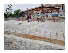
Asked to create a temporary bus depot site in Marseille for RTM, GCC Provence's Travaux teams and GCC's Technical Department seized the opportunity to launch a series of tests on the strength, durability and behavior over time of Hoffmann Green Cement Technologies' first H-UKR concrete made with Neolithe recycled aggregates. The target element for the test is the fuel loading bay slab of the depot.
