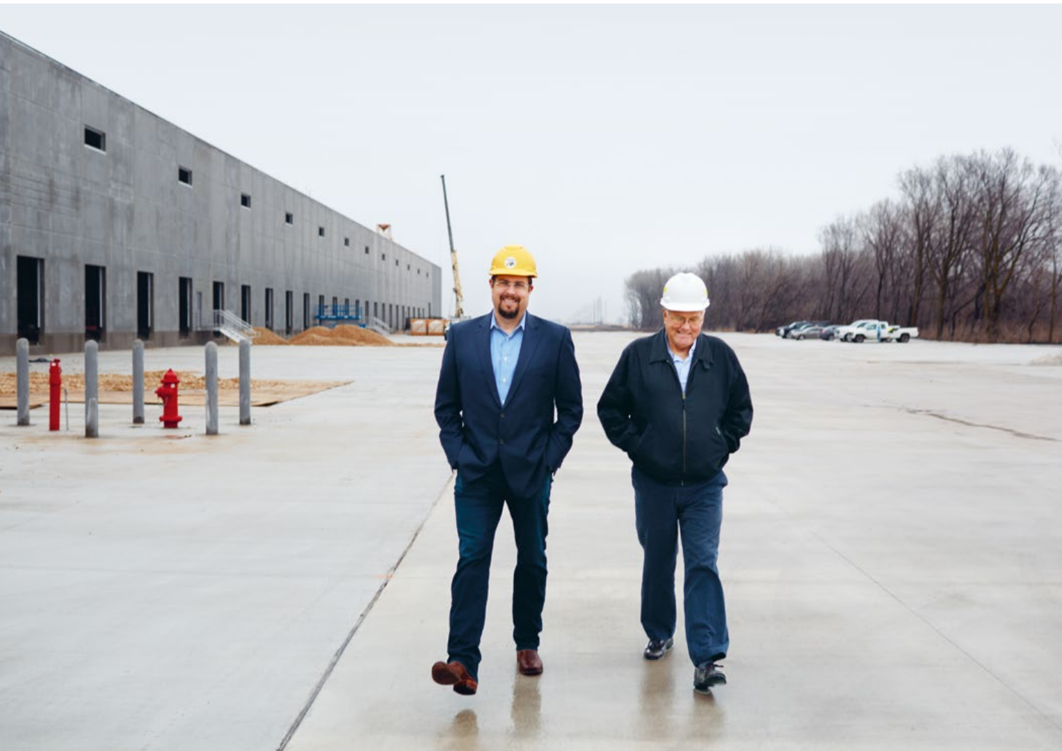
Jonathan Pease of Rock Solid and Tom Kiernan of LafargeHolcim at the job site in Channahon, Illinois.
