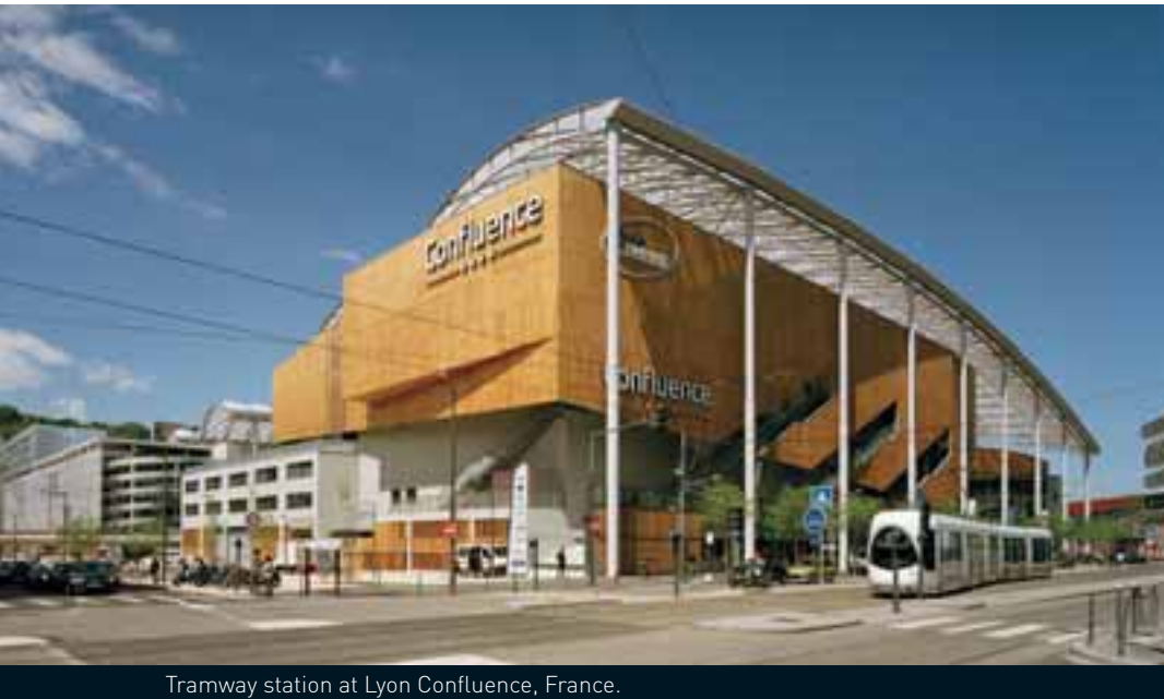
Tramway station at Lyon Confluence, France.
