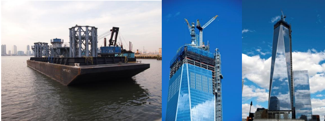
The finishing touch to One World Trade Center: the spire with tubes from Vallourec
