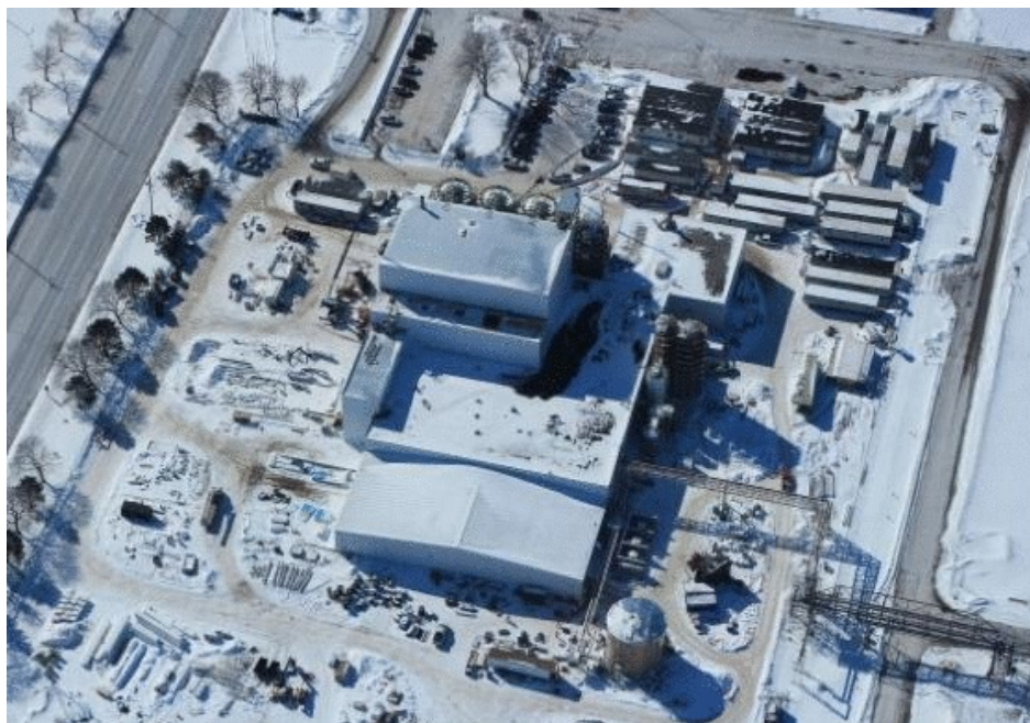
(Sarnia facility under construction)
