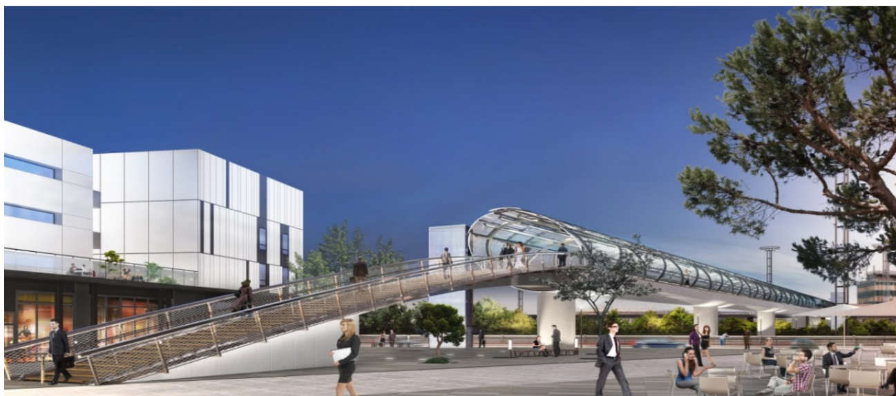
The footbridge as seen from the esplanade in the Cœur d'Orly business district © Groupe ADP
