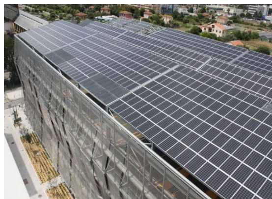
Silo de Parking – 230 kWc
