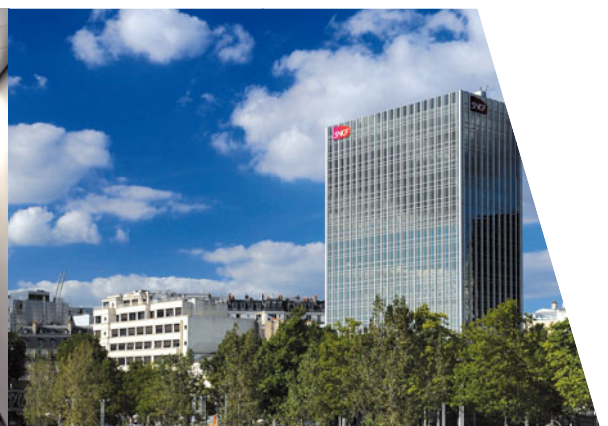
> Tour Traversière, Paris 12 e
