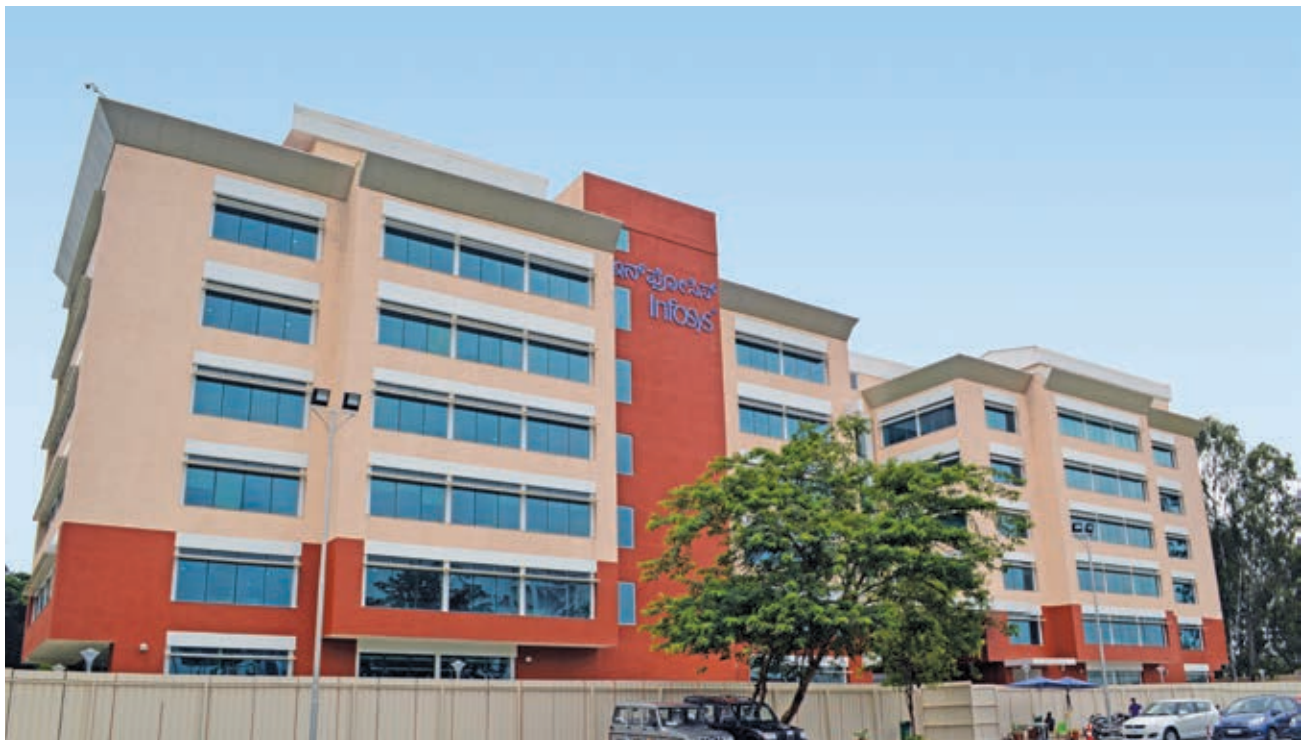
The LEED India Platinum-rated building in Bengaluru
