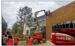
Construction du Shopping Promenade® de Claye-Souilly
