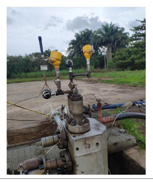
"Remote natural gas installation in Nigeria is monitored with a LoRaWAN® network using equipment from SRETT and Kerlink. Temperature and pressure data are sent to the owner's control room in near real-time, which eliminates the need for employees to travel to remote locations to check the equipment."
