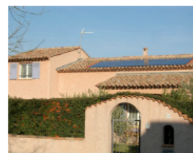
Installation Solaire Direct
