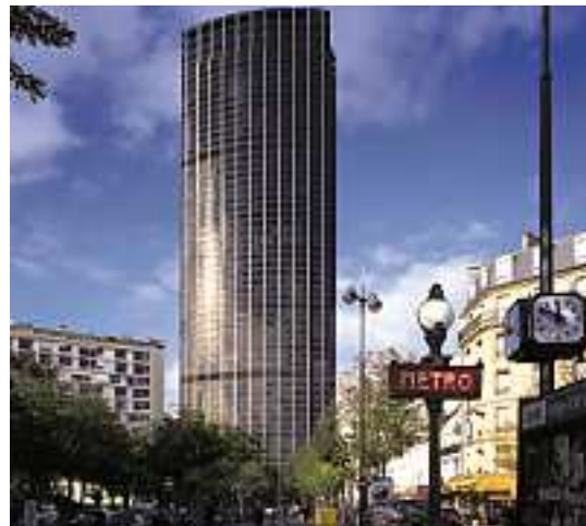
Ensemble immobilier Tour Maine-Montparnasse, Paris 15 e
